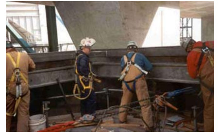
MRU Site Assembly # APEX USA
